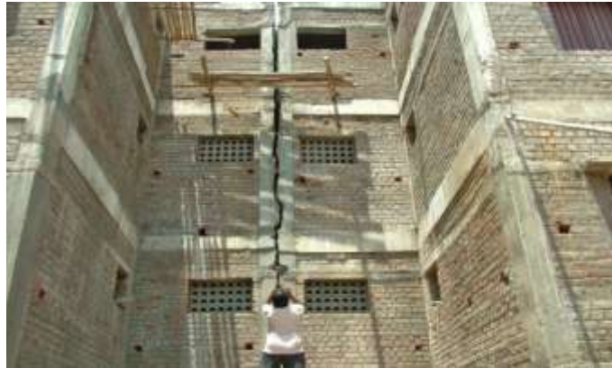
Figure 4. Crack in Expansion Joint Due To Settlement
