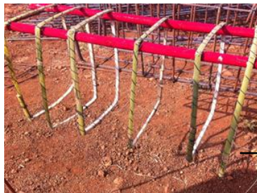
Fig. No. 5 Main and Shear reinforcement
