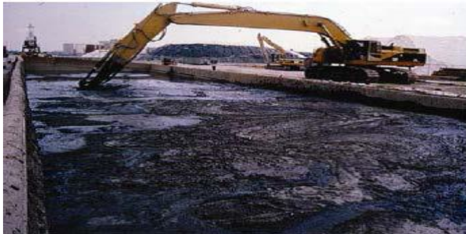
Ex-situ for on-site use stabilization (mixing in place of contaminated dredged materials)
