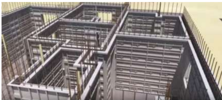
Fig. 1 Erected formwork for walls in monolithic construction
