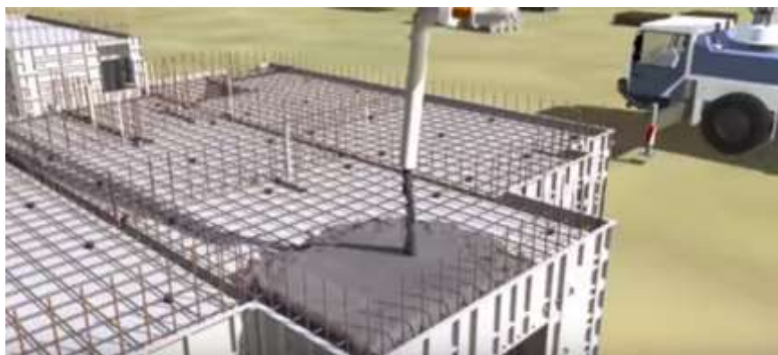
Fig. 2 View showing pouring of Concrete in to erected forms
