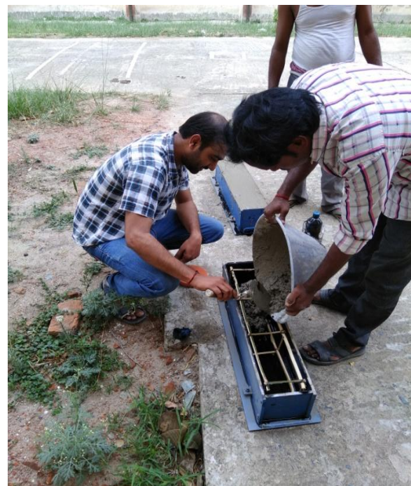
Fig. 4. Casting of beam Size 15cm x 15 cm x 70 cm
