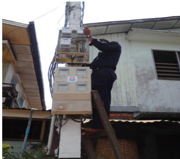
Fig 5 Installation of 1 Phase 2 Wire Offsite Meters Mounted on a Pole (with YESC Permission)
